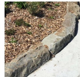
Example of how sandstone is used to frame raingardens
